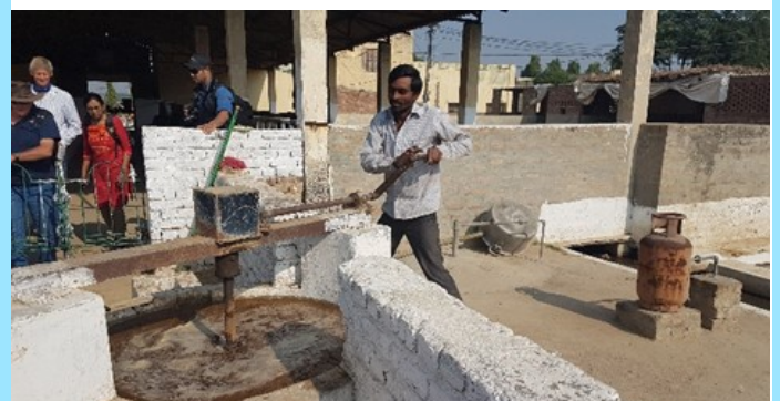
Preparation of cattle manure and urine to send to the digester. This will be added to the irrigation water to fertilise the fields.
